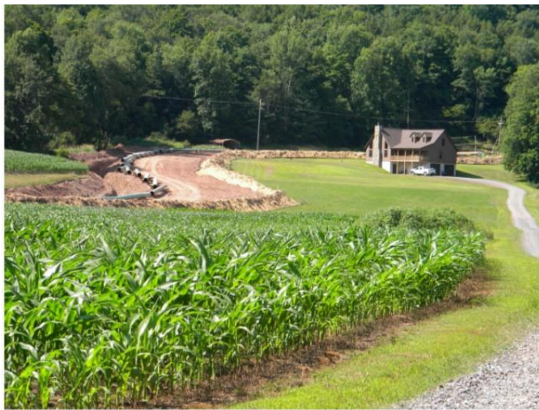
Gas gathering pipeline under construction near Warrensville, Lycoming County
